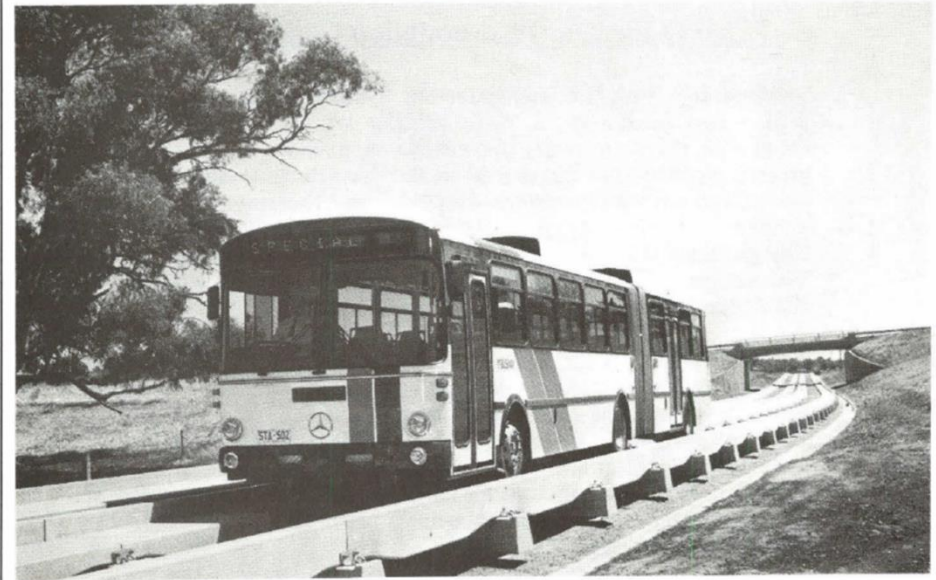
Fig. 2.1a The NorthEast Busway Adelaide - Australia
